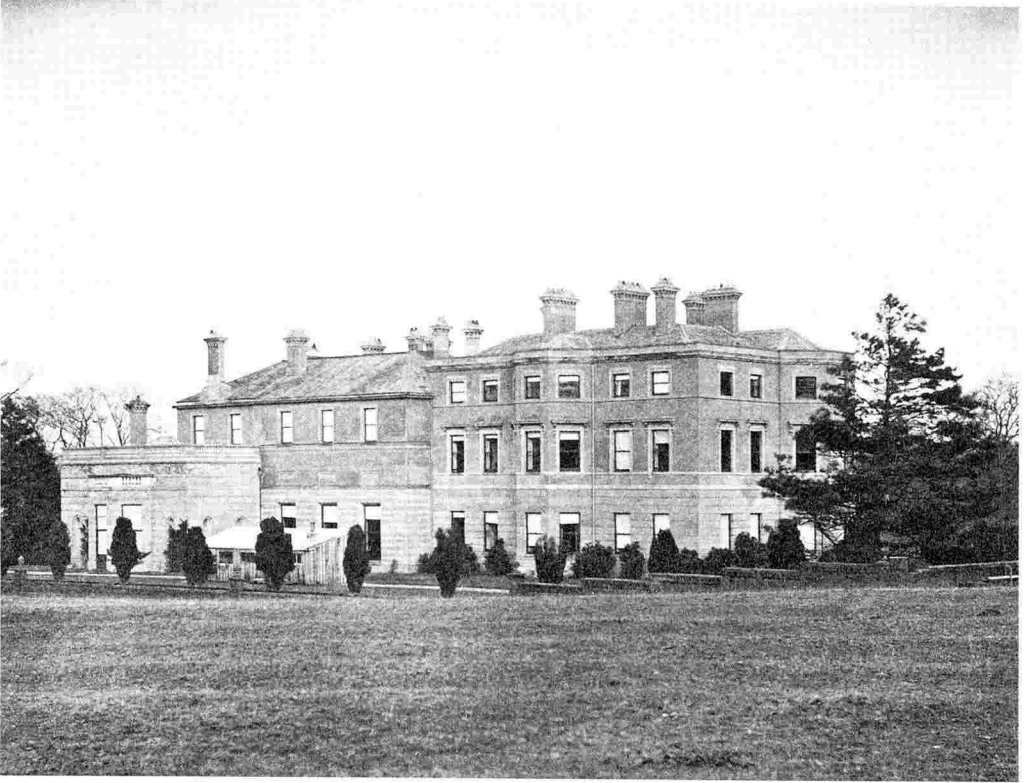
FIG. 26 – The south front of Riby Grove, Lincolnshire, birthplace of George Tomline, showing (left) the extensions carried out by the Bishop of Lincoln for William Edward Tomline (by permission of Mrs. M. Bence-Jones and the Suffolk Record Office).
